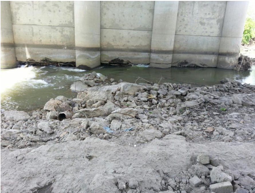
Look June 14th 2019 at stream flow diverted underneath center pier concrete wall of Martin Luther King (US150) bridge over North Fork River). Communicate and remedy condition.
