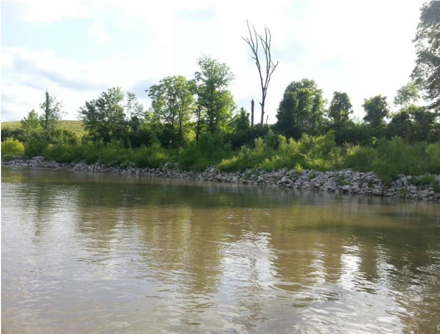
Look at rip-rap along the bank of Middle Fork River near deactivated power plant June 22nd 2019
