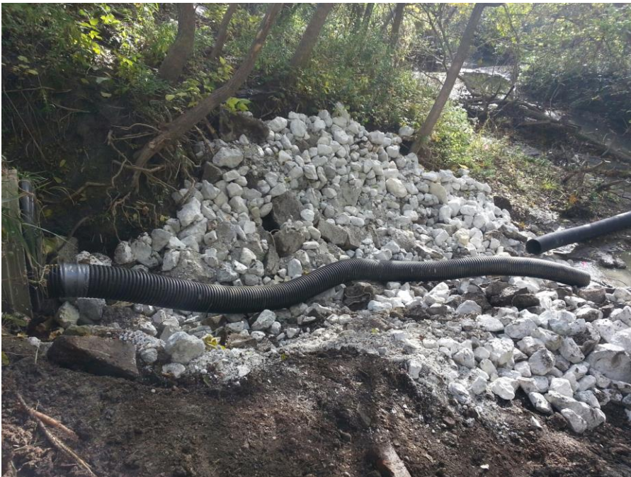
Look October 23rd at temporary bypass installed in 36 inch diameter storm sewer prior to grouting riprap
