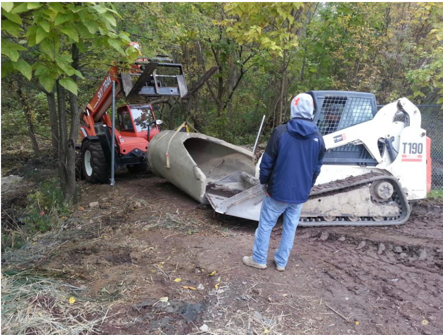
Look October 24th 2019 at sky track and tracked skid-steer dragging concrete flared end section 36 in diameter through fence
