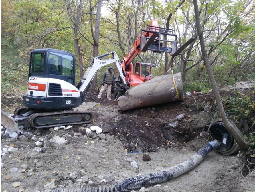
Look October 24th 2019 at mini excavator and fork lift handling and maneuvering 36 in diameter reinforced concrete flared end section for reuse at storm sewer discharge
