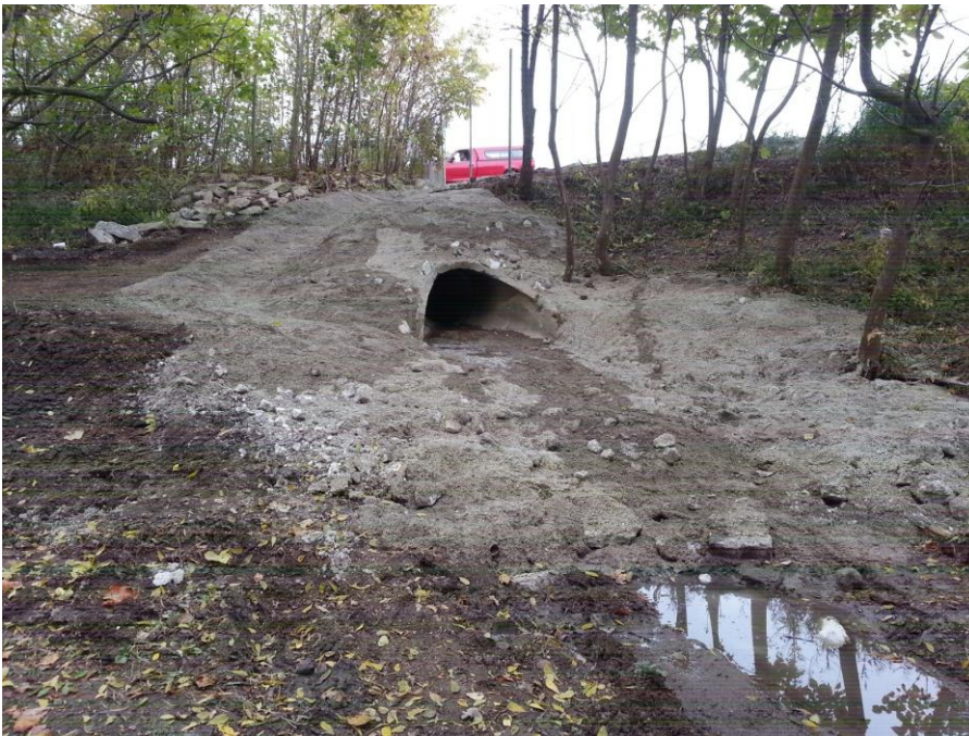
Look October 25th 2019 toward the northeast at the status of discharge and drainage swale riprap and concrete shape status at end of work day after temporary by-pass piping removed in anticipation of precipitation
