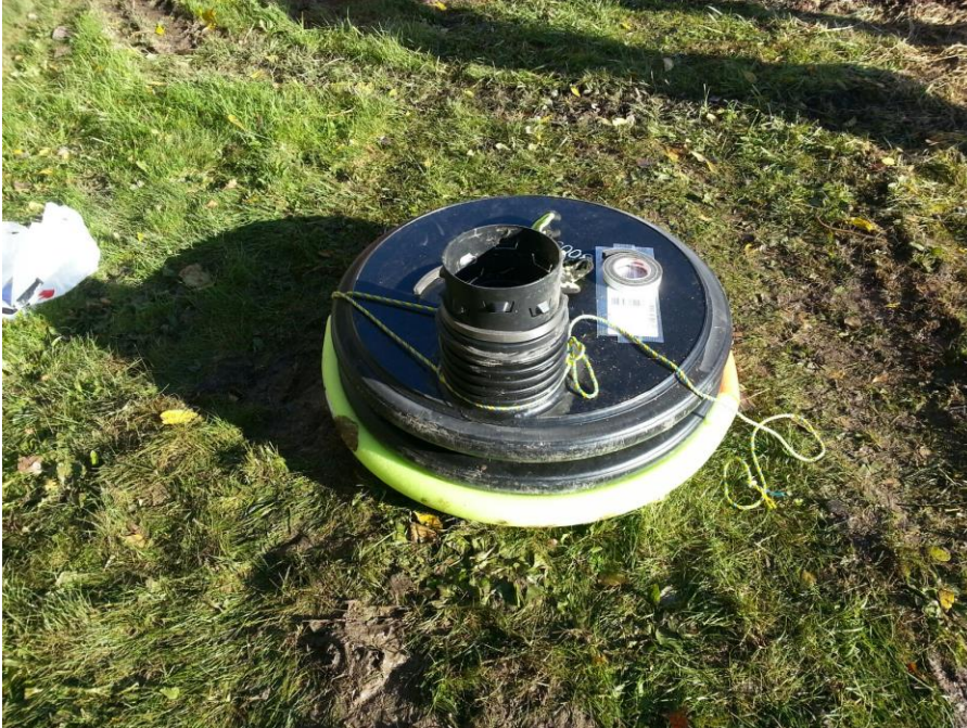
Look at temporary by-pass fitting prior to installation into storm sewer pipe October 23rd 2019
