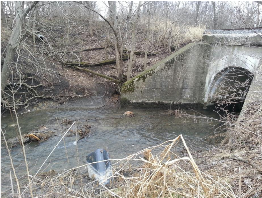
Look southwesterly at arch concrete bridge structure at CSX railroad over branch of Grape Creek. Notice storm sewer discharging from bank. Water is bleeding from behind abutment. Photo taken January 23rd 2020
