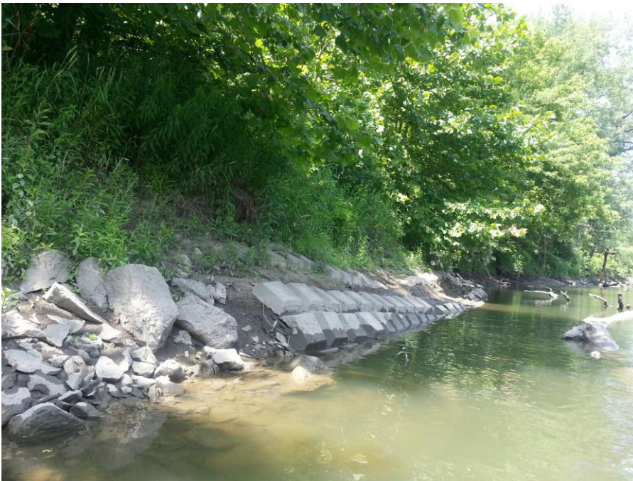
Look westerly July 24th 2019 at condition of concrete revetment mat along south bank of Vermilion River approximately 100 to 200 yards upstream of the Tilton Arch CSX Railroad Bridge near General Motors site
