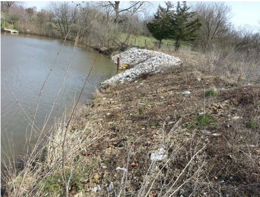
Look southeasterly at screened culvert inlet and dam on Herschel Lake April 10th 2019. Coordinate with Engineer to establish vegetation and prevent erosion of exposed soil.
