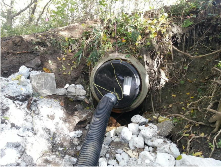
Look at temporary bypass fitting installed in 36 inch diameter storm sewer prior to riprap grouting
