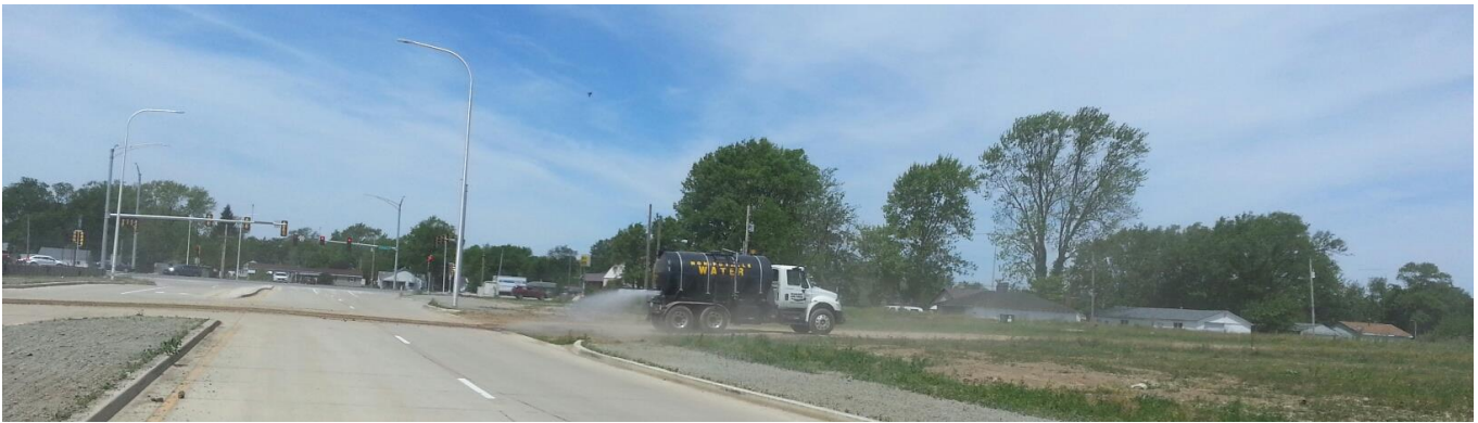
Look west June 14th 2019 at water truck being utilized to control dust along haul road for earth-moving operation.
