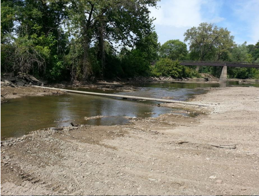
Look northerly September 13 th 2019 from east bank of North Fork River at pipe exposed across North Fork River. Determine purpose of pipe and eliminate hazard.
