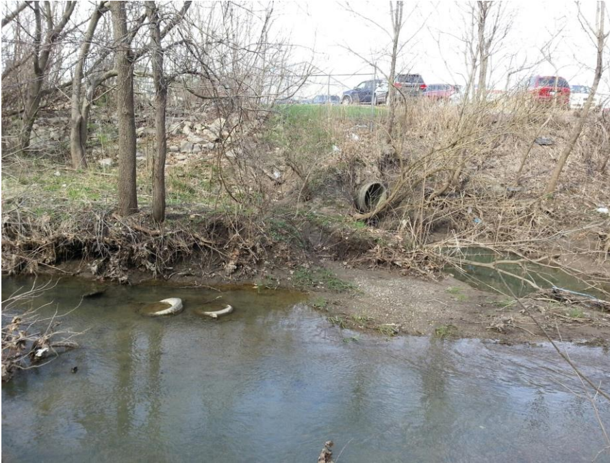
Look towards Northwest at erosion near 36-inch Southgate Drive storm sewer discharge April 10th 2019 from the south side of Grape Creek. Remove tires from stream and coordinate with Army Corp of Engineers requirements according to Nationwide Permit 7.
