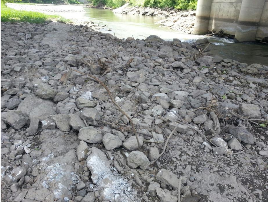
Look June 14th 2019 at reinforcement-bar protruding from concrete debris under Martin Luther King (us-150 Main Street Bridge) on North Fork River east of center pier
