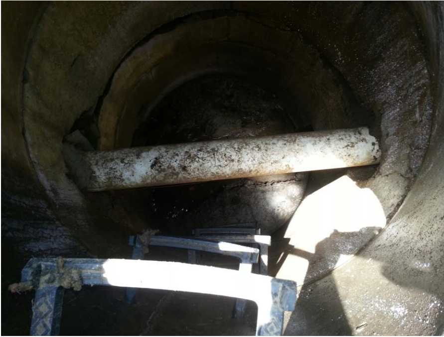
Look May 22nd 2019 in Storm Sewer Manhole C8 at possible conflict sanitary line in storm sewer manhole
