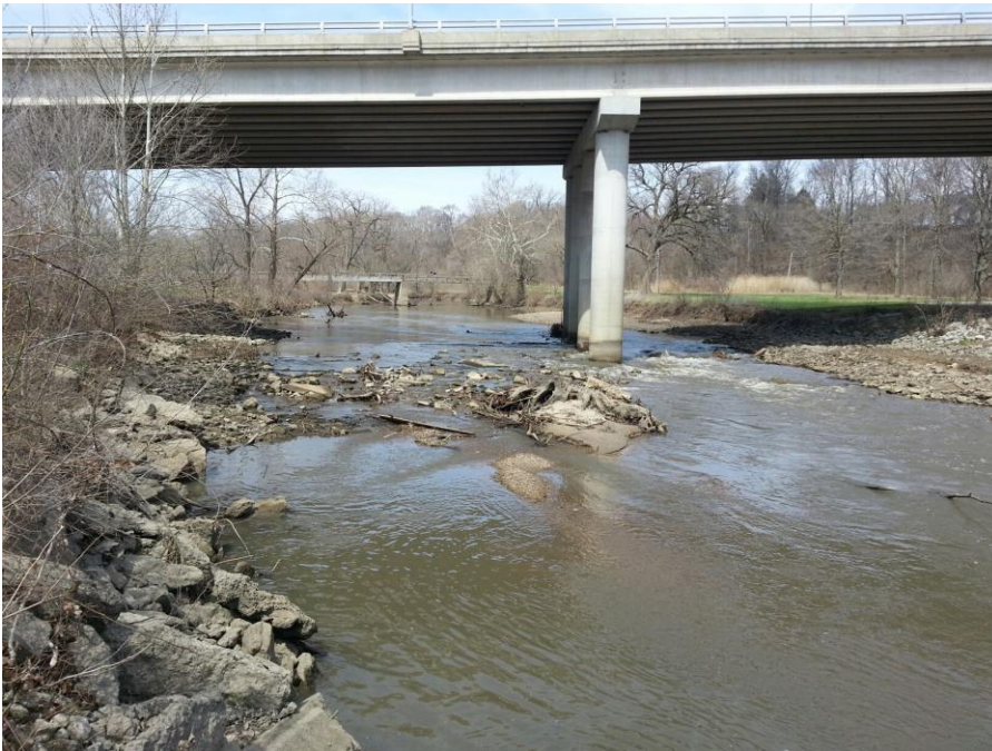
Look April 6th 2019 from the west bank of the North Fork River upstream of dam removal project in Ellsworth Park at the U.S. 150 Bridge over the North Fork River. Water flowing towards and under center pier also demolition debris exposed due to lower water elevation. Remedy conditions.
