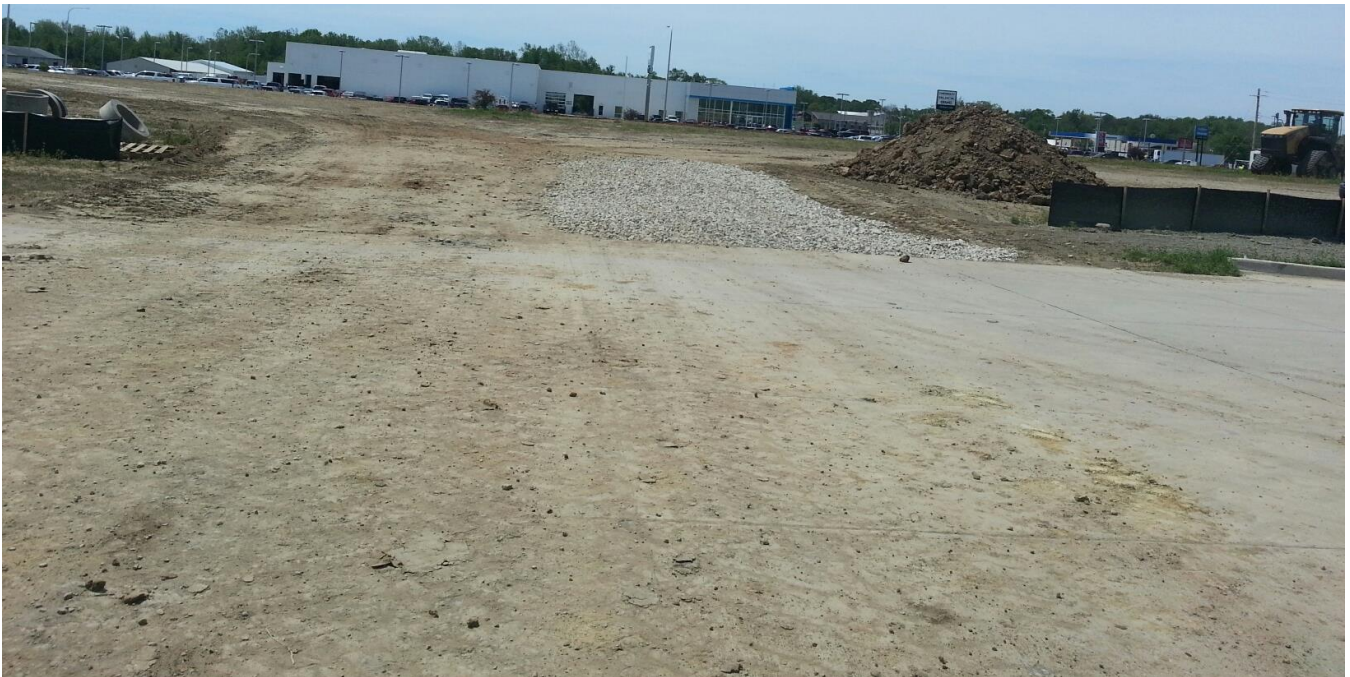
Look southerly June 14th 2019 at stone construction entrance placed on the north side of Mach1 site. View is from Ramp Road.
