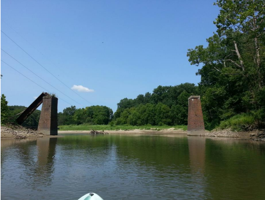
Look towards upstream along Vermilion River at brick piers and steel structure collapse July 24th 2019. Determine owner of structure.
