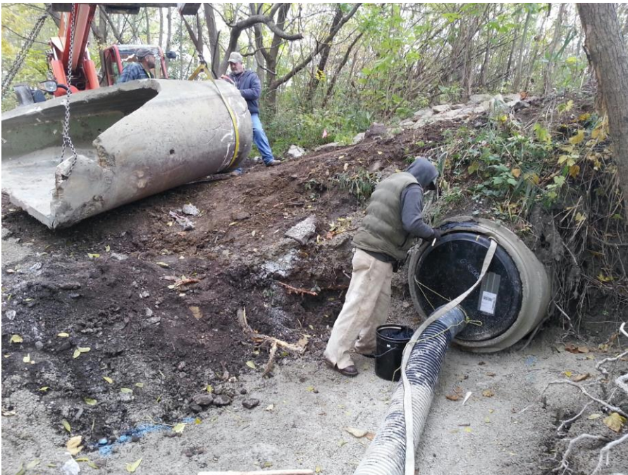
Look October 24th 2019 at mastic placed at joint prior to flared end section being installed on 36 inch diameter storm sewer discharge
