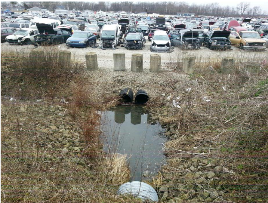
Look January 23rd 2020 toward downstream at two 24 inch diameter HDPE culvert under automotive salvage yard
