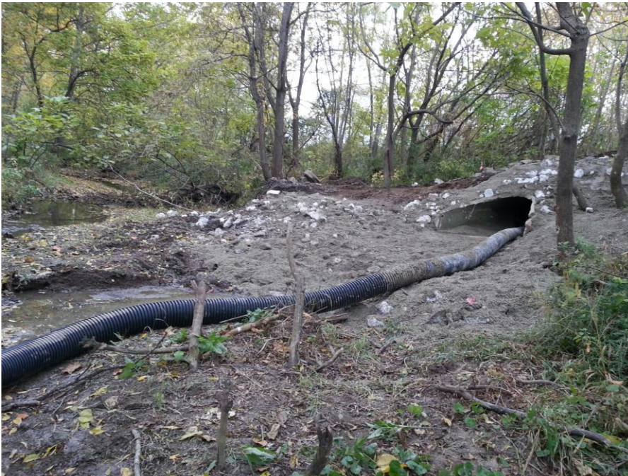
Look October 24th 2019 towards the northwest at status of end section repair and dissipation riprap grouting at end of work day
