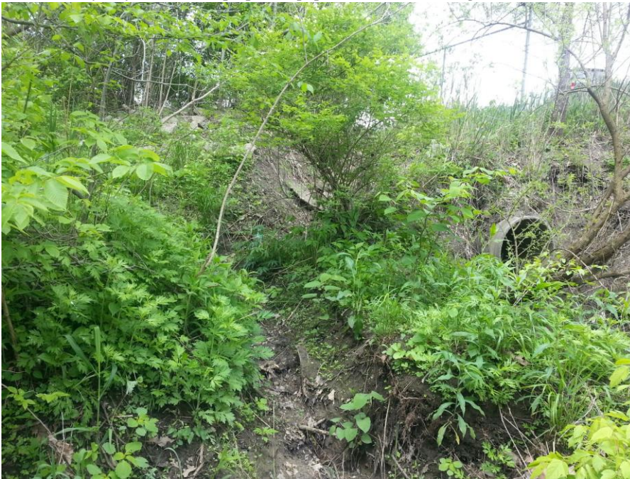
Look northerly May 13, 2019 at erosion rut proposed for fill with riprap grouted from the top to the bottom may minimize required vegetation clearing to access storm water discharge.
