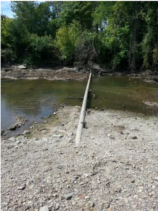
Look September 13th 2019 at pipe line across North Fork River exposed upstream of us 150 Martin Luther King Drive Bridge. Dam removals exposed hazard. Communicate to determine pipe owner and eliminate hazard of exposed pipe obstructing water way.
