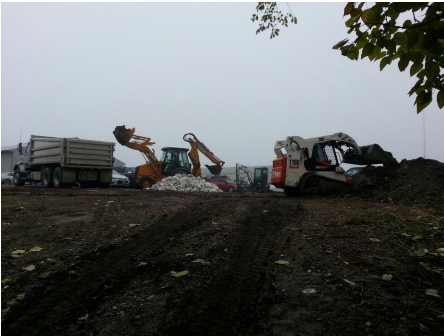
Look northeasterly October 28th 2019 at wheel loader backhoe, tandem dump truck and rubber track skid steer being utilized to during site restoration effort
