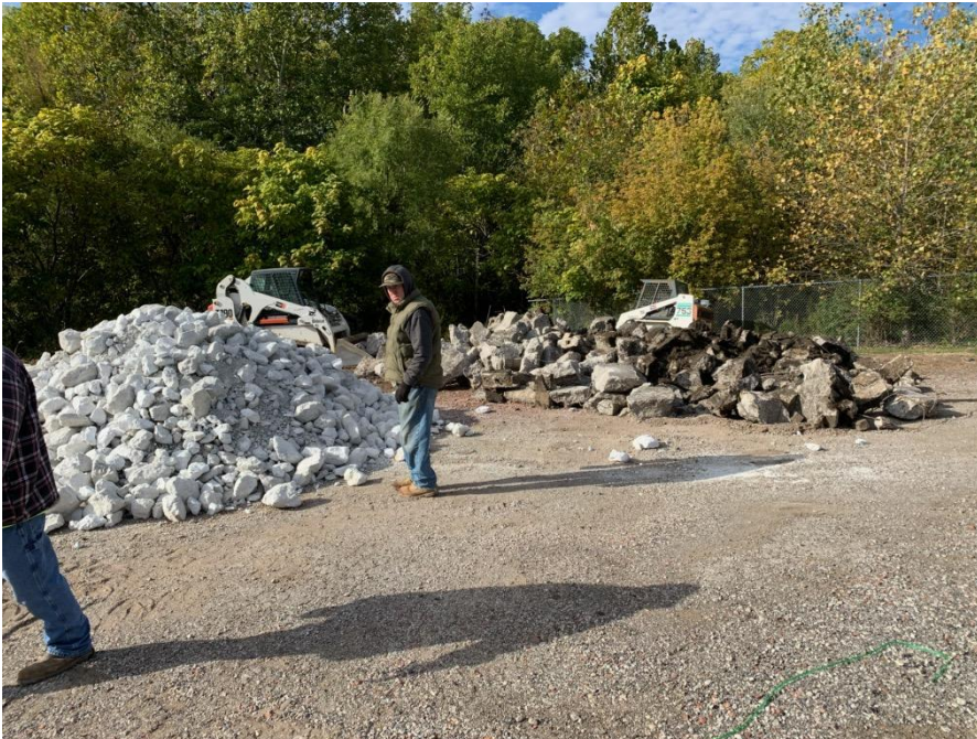
Photo provided by Offutt of recycled rubble concrete and stone rip rap stockpiles site prior to placement
