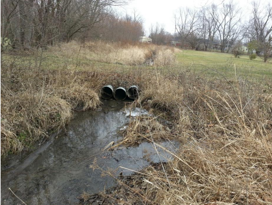
Look toward east at 3 corrugated metal culvert pipes under access path January 23rd 2019 upstream of WITY radio tower
