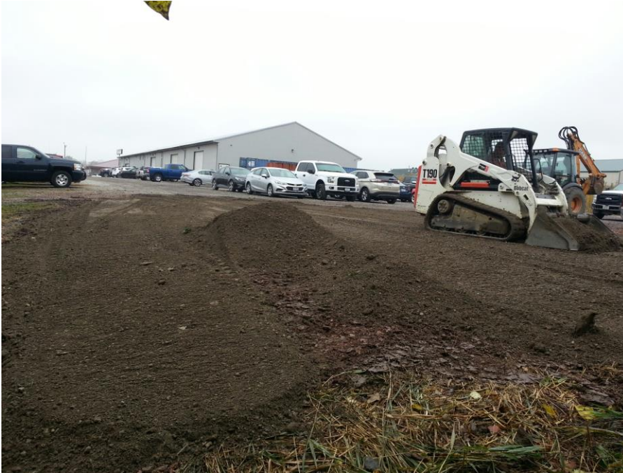
Look northeast October 28th 2019 at rubber tracks skid steer grading a load of crushed recycled concrete on disturbed auto body repair facility parking area
