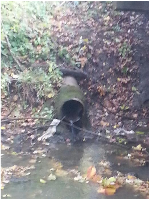
Look northerly October 21st 2019 at storm sewer discharge near the northwest corner of King Street Bridge over Grape Creek. Notice material restricting flow during previous inspections removed.
