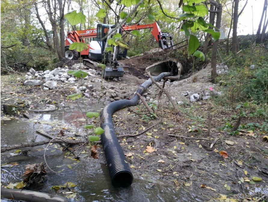
Look northerly October 24, 2019 at 36 inch diameter concrete flared end section, temporary bypass pipe and equipment while in propped and leveled into position on riprap prior to grouting operation
