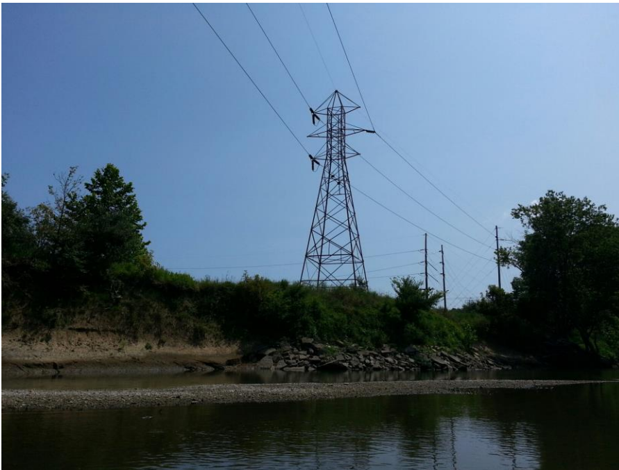
Look toward downstream on Vermilion River July 24th 2019 at overhead utility structures. Communicate with utility company to inspect condition of bank near structures to ensure structural stability. Give notice to Army Corps of Engineers to obtain permission prior to discharge of erosion stabilization material onto bank
