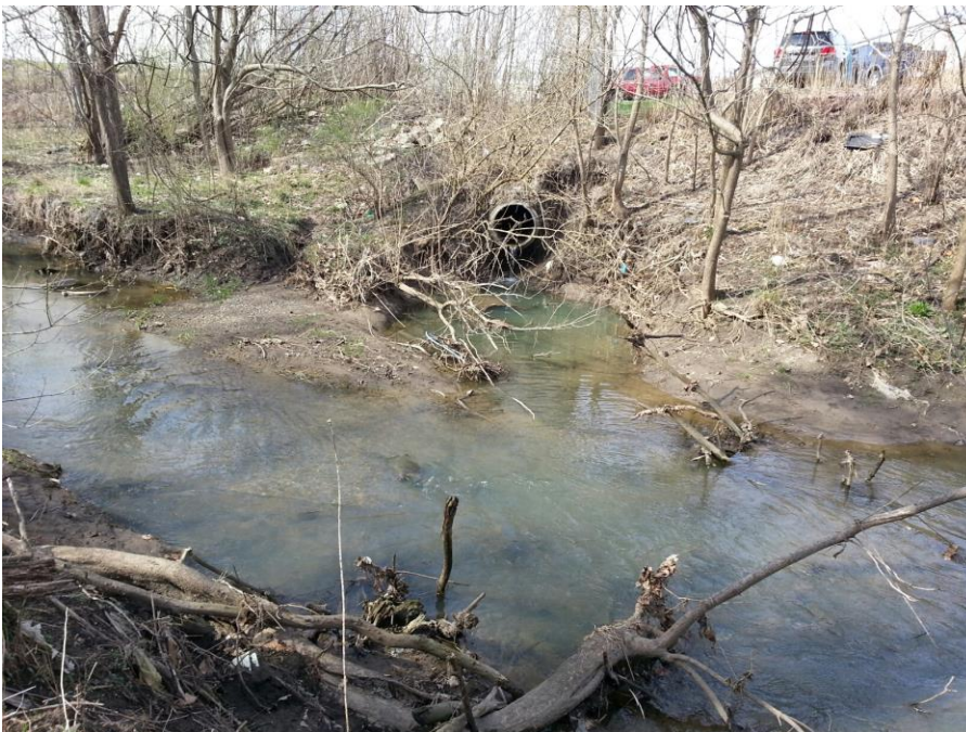
Look April 10th 2019 from the south side of stream towards the north across Grape Creek at erosion near 36 inch diameter storm sewer discharge from Southgate Drive. Coordinate with Army Corp of Engineers requirements according to Nationwide Permit 7.
