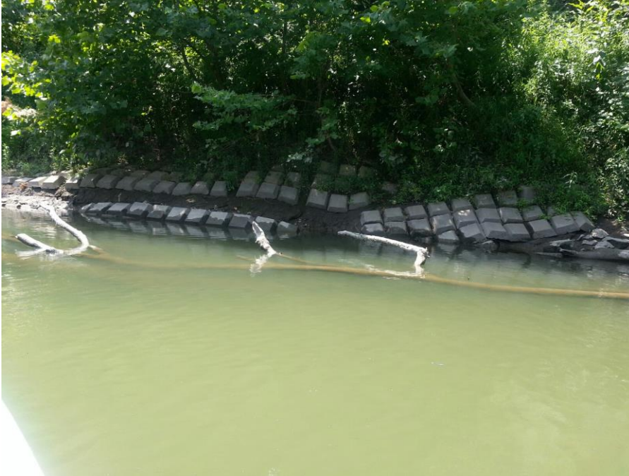
Look south at exposed concrete revetment along bank near General Motors site upstream of Arch CSX Railroad bridge July 24th 2019
