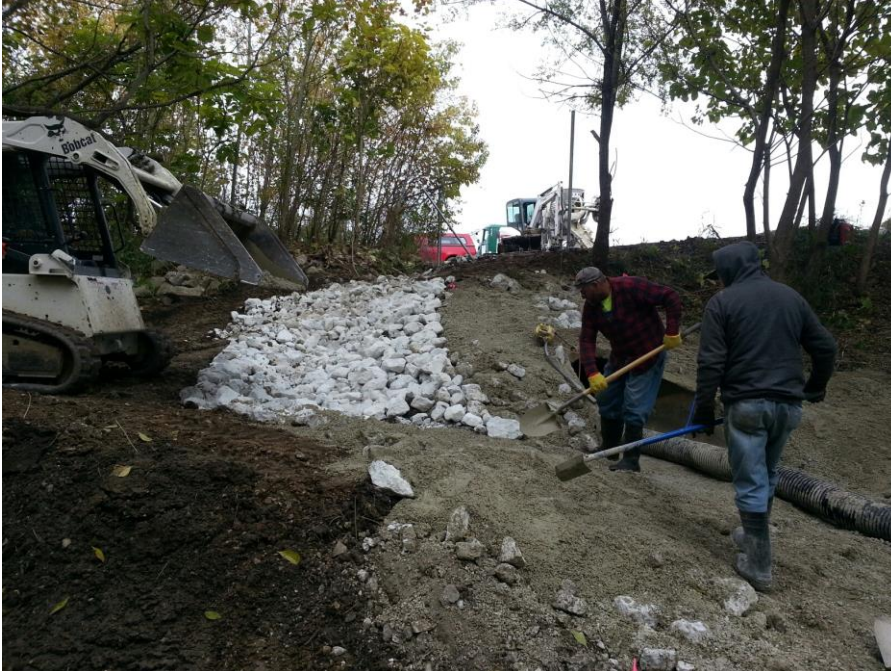
Look northeast October 25th 2019 at crew mixing grout into graded riprap drainage swale voids
