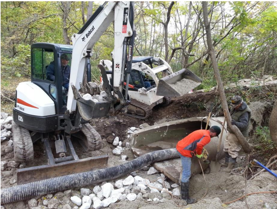
Look October 24th 2019 northwest at concrete and riprap mixing with vibrator, manual shoveling, mini excavator placing rip rap and skid steer delivering cement aggregate mix around flared end section to stabilize and anchor
