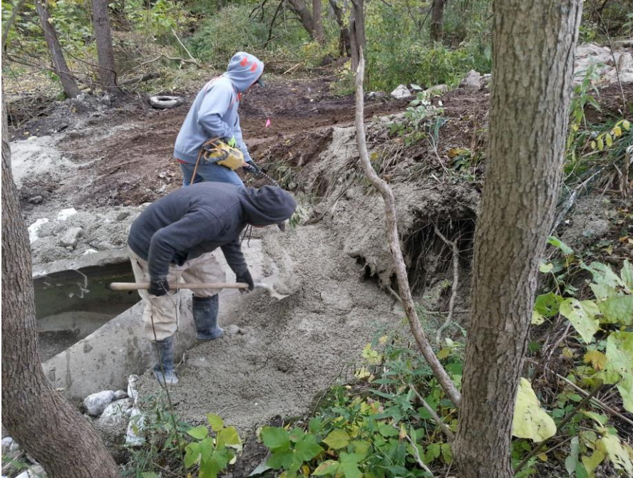
Look October 24th 2019 at concrete collar being placed on the exterior joint of flared end section and storm sewer pipe
