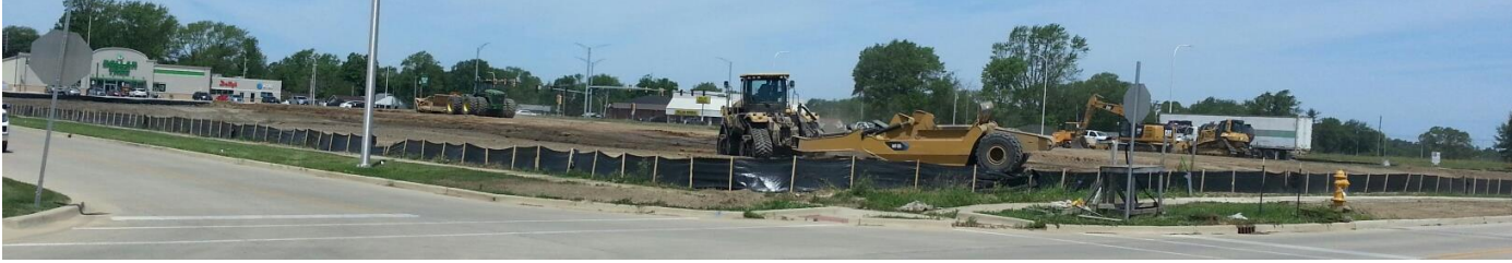
General view toward Northwest June 14th 2019 from the intersection of First Avenue and 16th Street at Mach 1 fuel station site at scraper hitched tractors grading and silt fence installed around the perimeter.
