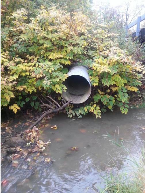
Look south October 21st 2019 at pipe near the southeast corner of King Street Bridge over Grape Creek. No water observed discharging from pipe after rain events. Consider robotic video inspection of pipe.
