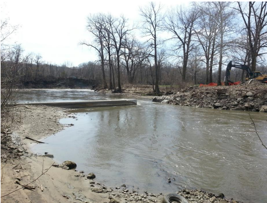
Look southeasterly from east bank of North Fork River at Ellsworth Park Dam removal status April 6th 2019. Safely remove tire and rebar immediately from drainage way and legally dispose of.
